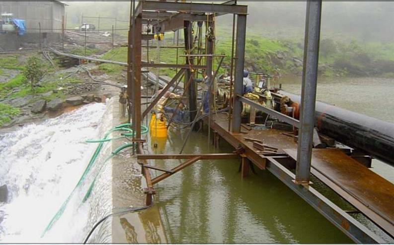
HEP's on non perennial rivers (especially those with many surrounding yet non - linked water bodies) can benefit from water harvesting - water from these reservoirs (which do not feed the turbine) is pumped to the main reservoir from where it shall feed the turbine thereby resulting in power generation.
